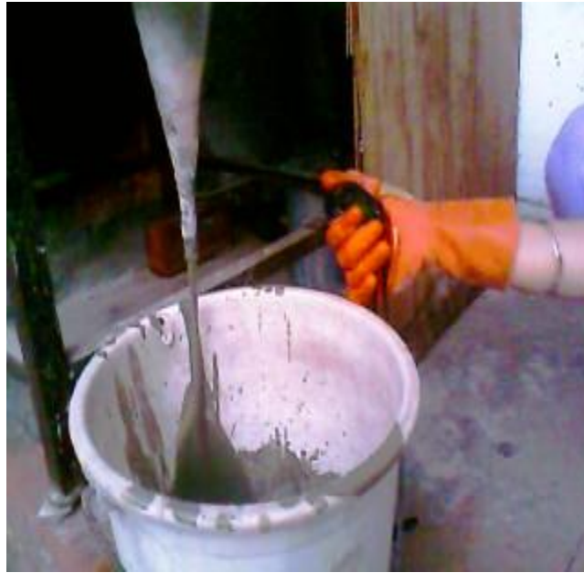
Fig 18 Flow of slurry after opening orifice
