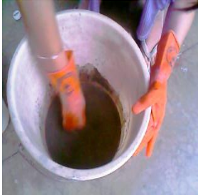
Fig 12 Mixing of Cement, SP and Water
