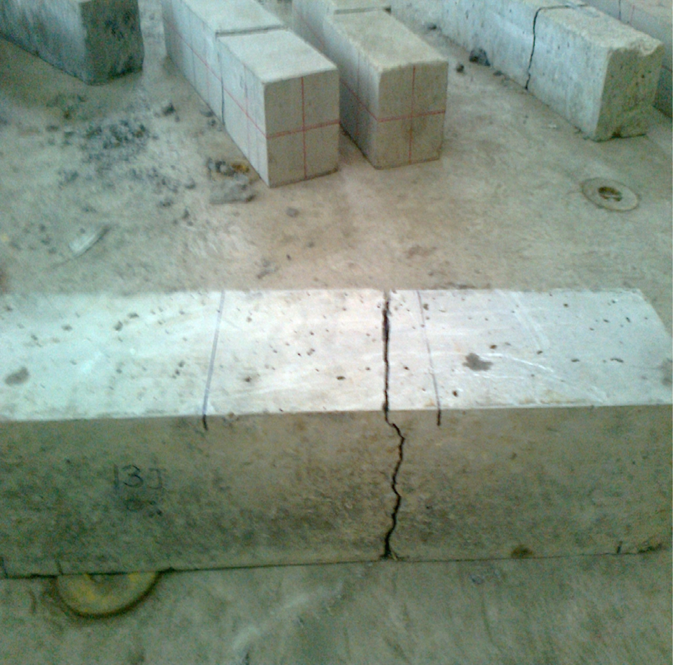
Fig 7: One of the concrete samples with no steel fiber
