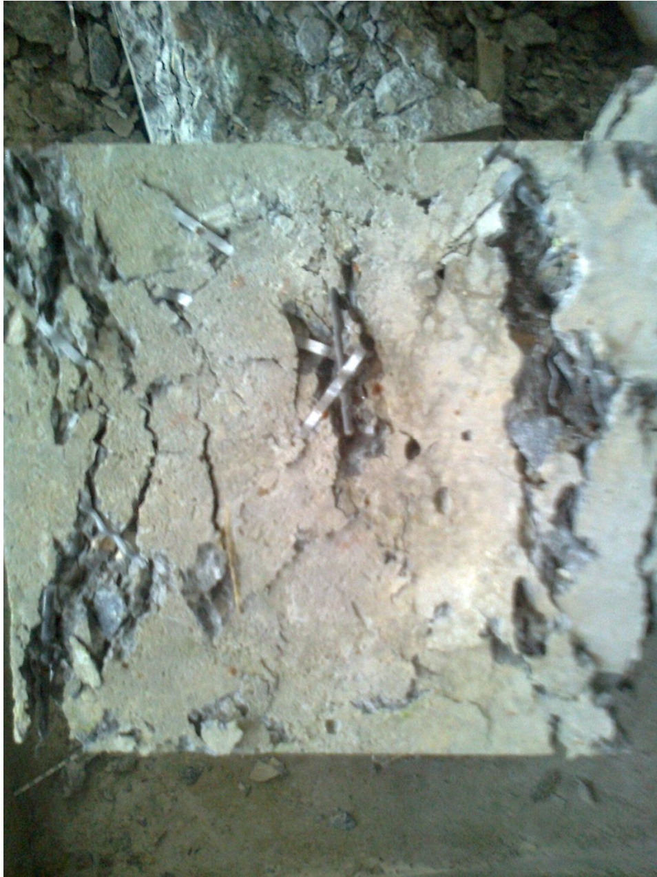
Fig 5: One of the concrete cubes with steel fiber after testing
