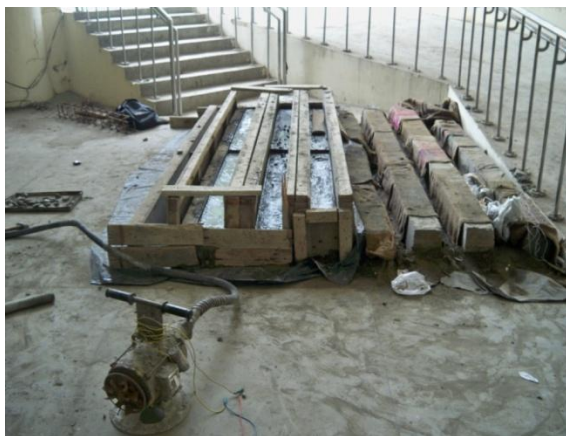
Fig 3.9: Casting and Curing of RCC Beams
