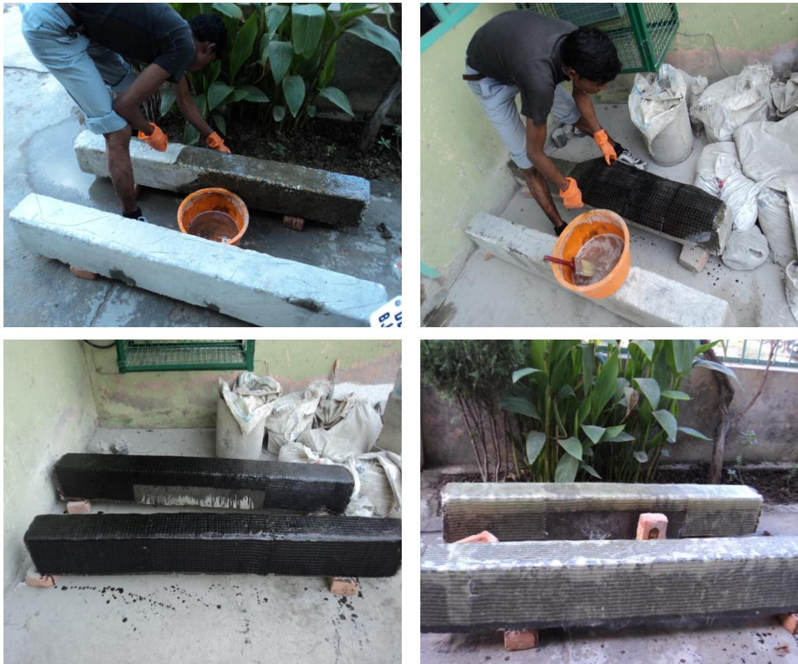
Fig 3.10: Application of FRP composites
