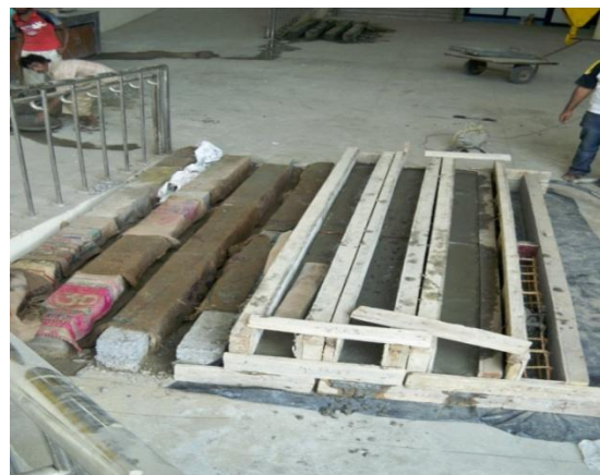
Fig 3.9: Casting and Curing of RCC Beams
