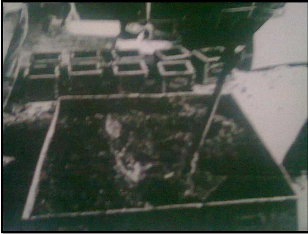
Fig 3.1 Mixing of materials.
