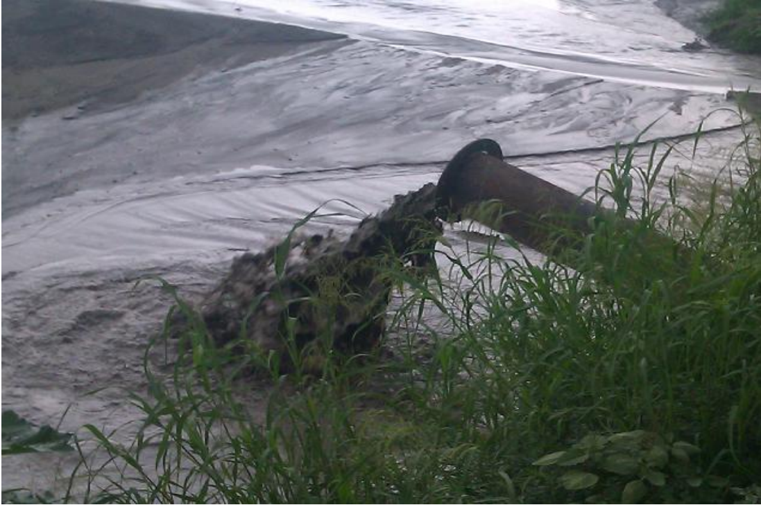
Pic. 4 - Wet disposal of pond ash from Rajghat Power Station
