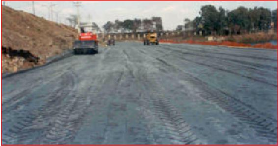
Pic. 2 - Construction of embankment with fly ash at second Nizamuddin Bridge in Delhi
