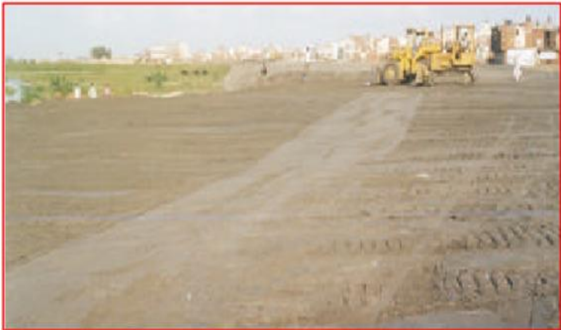
Pic. 2 - Construction of embankment with fly ash at second Nizamuddin Bridge in Delhi
