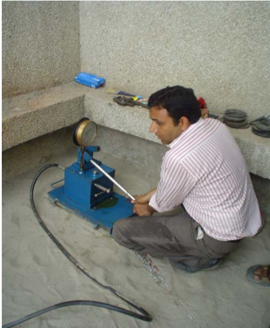
Fig 3.11:-Loading from hydraulic jack during testing
