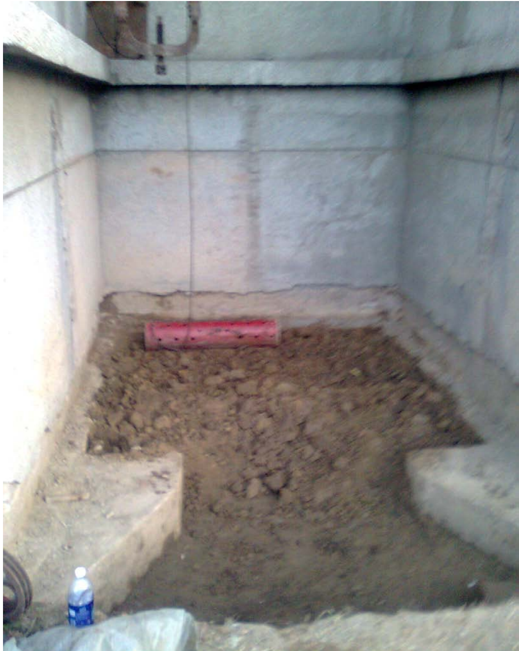
Fig 3.3:-Pit at Initial Stage
