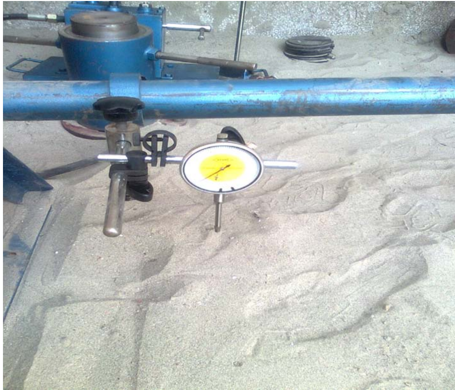
Fig 3.7:-Dial gauge arrangement on site
