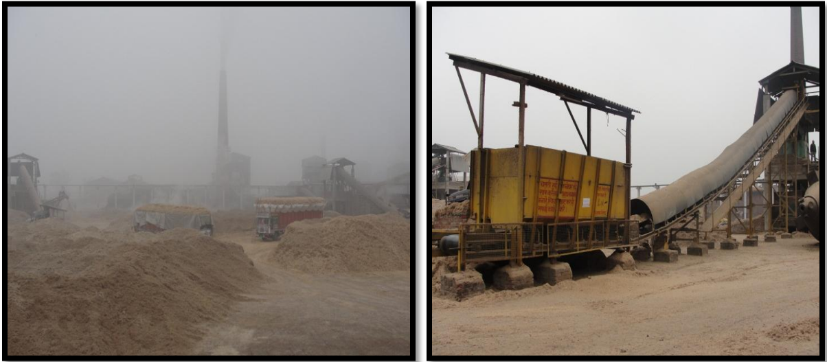
Figure 4.7: Raw Material Yard House
