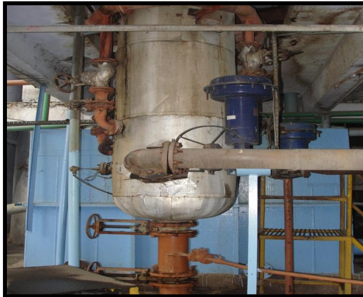
Figure 4.12: Closed Blow Discharger (CBD)
