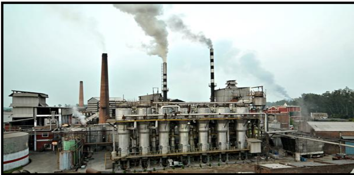
Figure 5.1: Soda Recovery Plant at Naini Tissues Ltd., Kashipur
