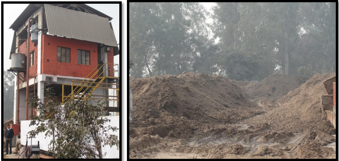
Figure 6.10: Sludge Thickener Facility and Sludge Storage Area
