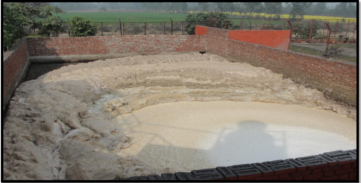
Figure 6.4: Foam Yard for collection of Bleaching Wastewater and Combined Wastewater from the manufacturing process
