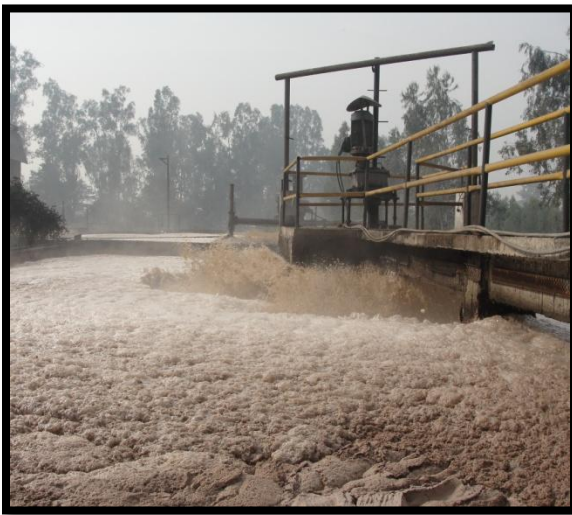
Figure 6.7: Aeration Tanks in Effluent Treatment Plant (Naini Tissues Limited)
