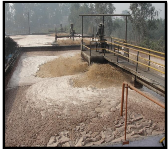
Figure 6.7: Aeration Tanks in Effluent Treatment Plant (Naini Tissues Limited)
