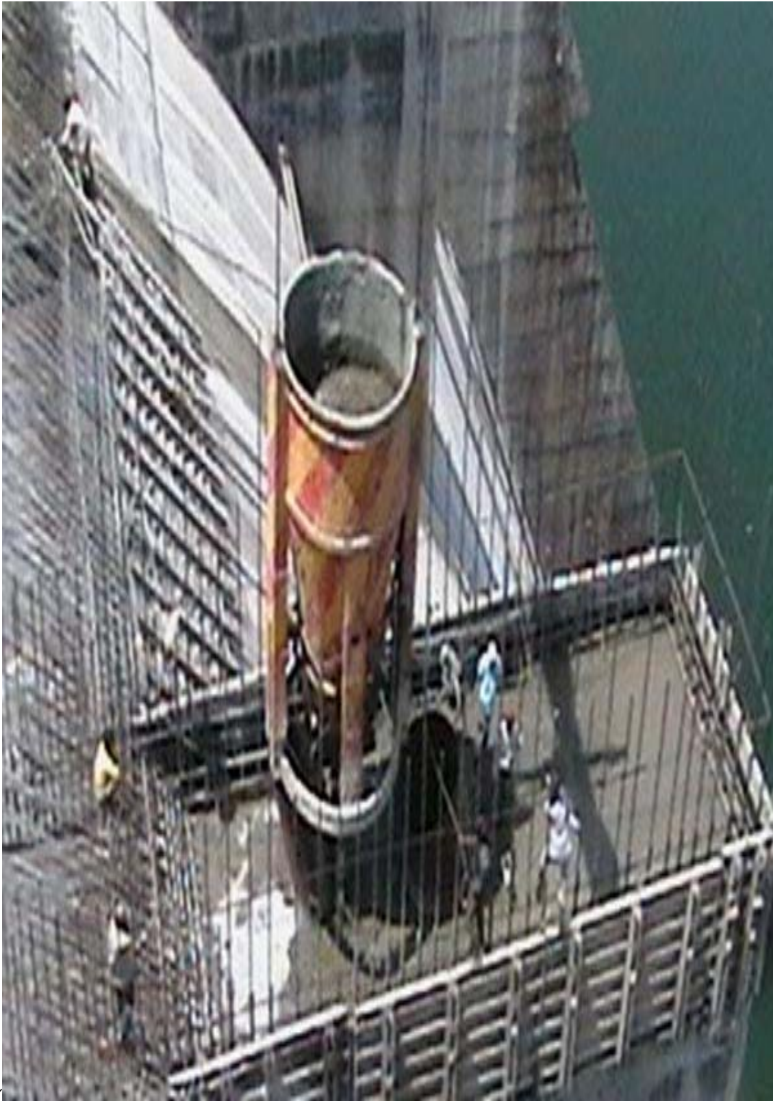
Fig 2.9 Today's photo of Navagam dam work
