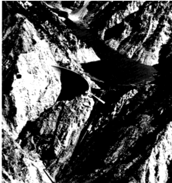
Fig2.3 Pacoima Dam, California, was subjected to 1971 San Fernando earthquake; the seismic motions were recorded by a seismograph on narrow rock ridge above the left abutment, at the point indicated (Courtesy of George W. Housner)
