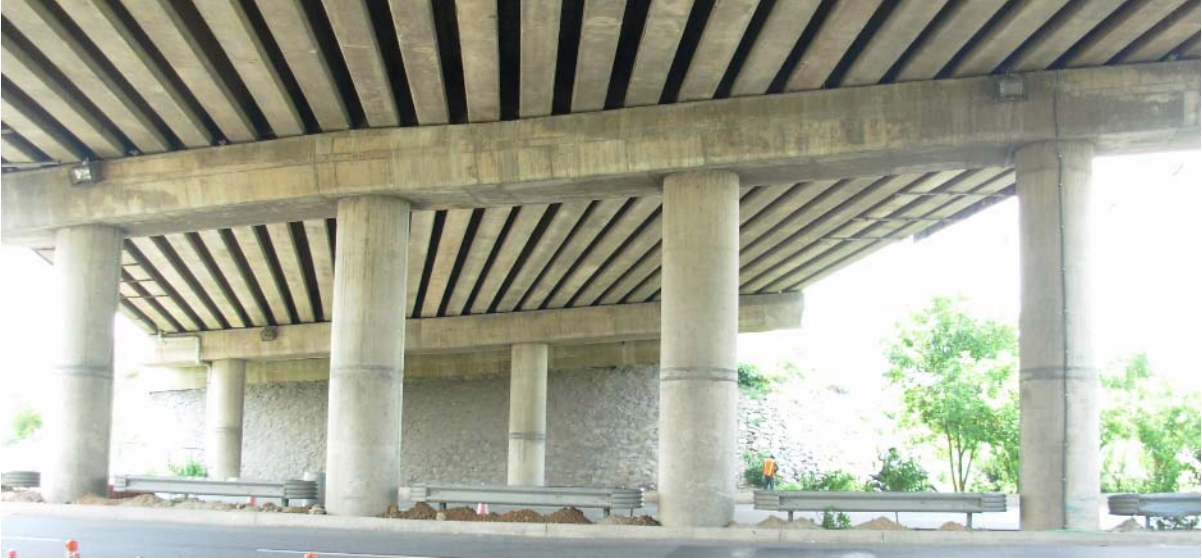
Fig. 4.7 Pictorial view of Bent beam-Pier system
