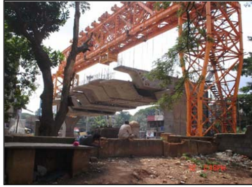
Erection of Box Girder Segments – Flyover at Anand Rao Circle.
