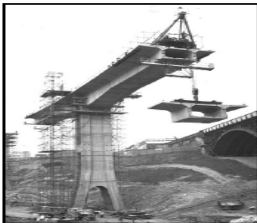
Fig. 1(a) : Erection of segments with shear leg segments through columns.
