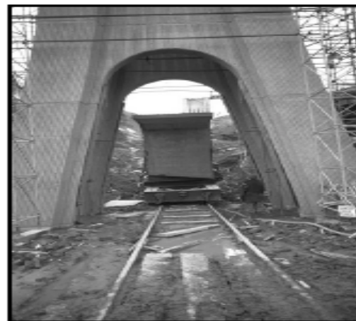
Fig. 1(b) : Delivery of segments through the piers.
