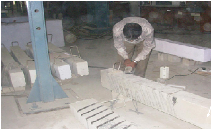
Fig 2.5 Grinding of beam surface at strengthened side to remove excessive mortar
