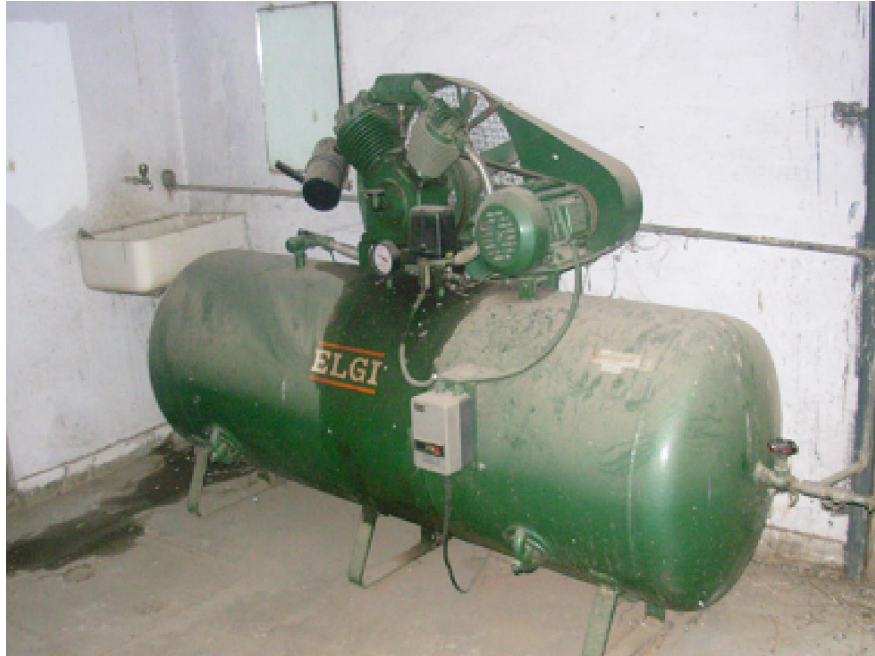
Fig 2.6 Air compressor used for cleaning the grooved surface
